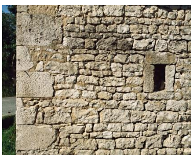
Bauernhofscheune Chézeaux in Douadic (Indre)
